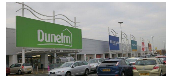
Park post refurbishment
